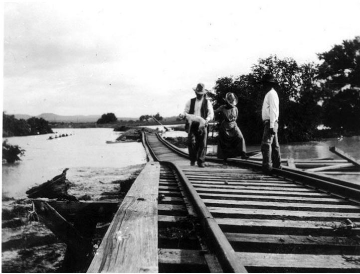
Flood damage at the Guadalupe River at Comfort, Texas, July 13-18, 1900 after heavy rainfall (image from www.floodsafety.com ).
