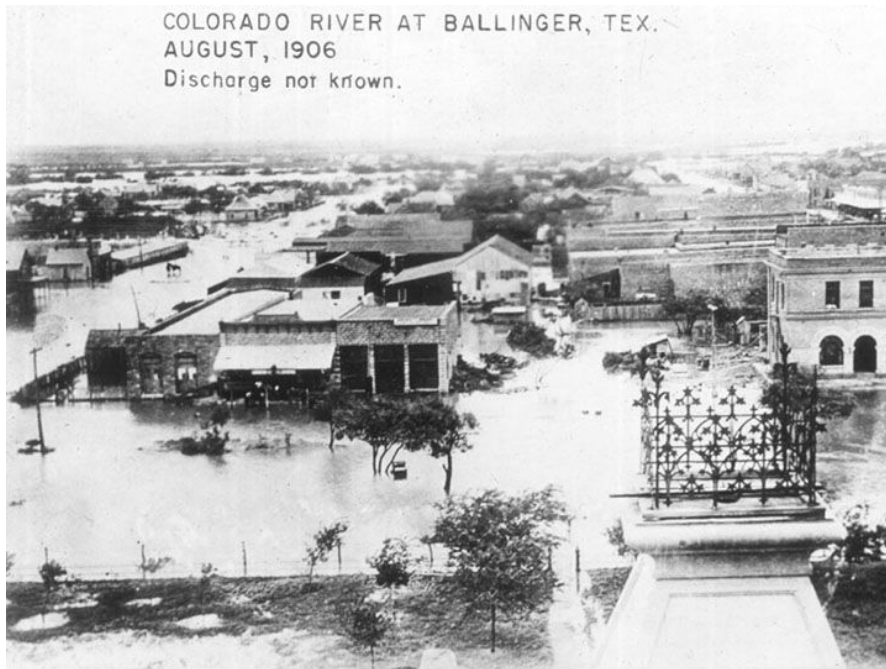
Flooding from the Colorado River at Ballinger, Texas, August 5-6, 1906 after more than 8 inches of rainfall occurred over the upper Colorado River basin (image from www.floodsafety.com ).
