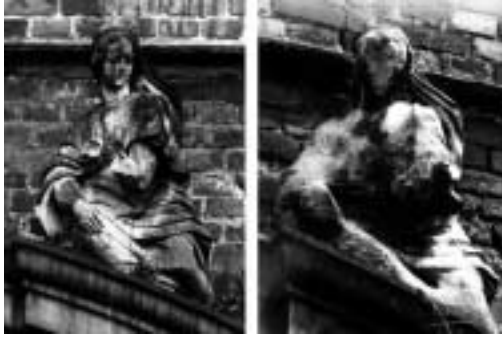
Figure 3.10x2 Acid rain damage to statuary, 1908 & 1968
